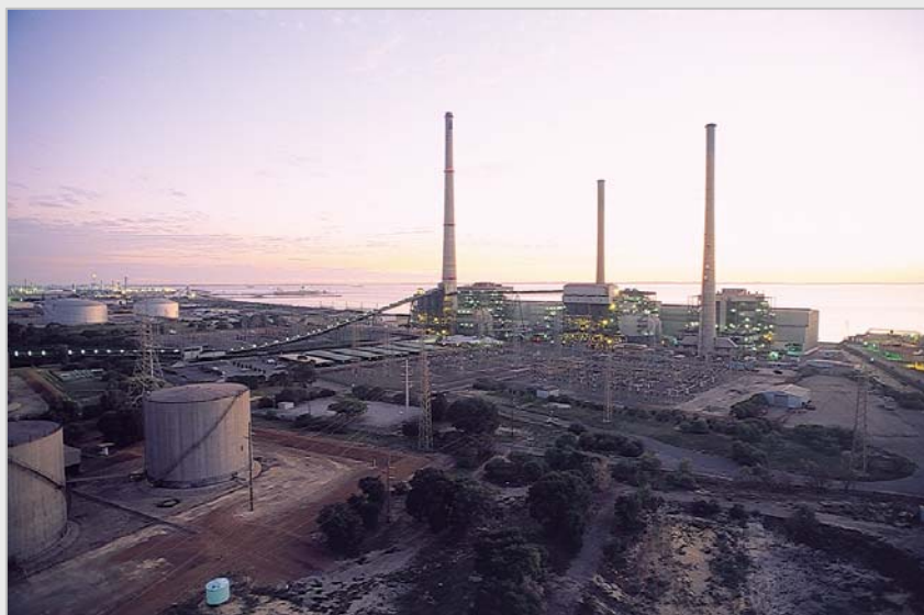
Photo courtesy of Western Power
